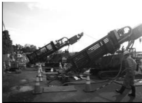
Figure 4. Inclined drilling in operation.
